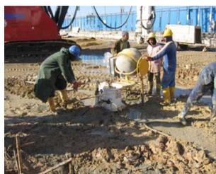
Post test grouting of a working pile
