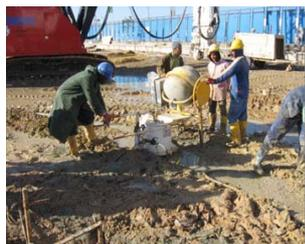
Post test grouting of a working pile
